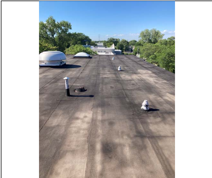
Modified Bitumen Roof, above Third Floor
