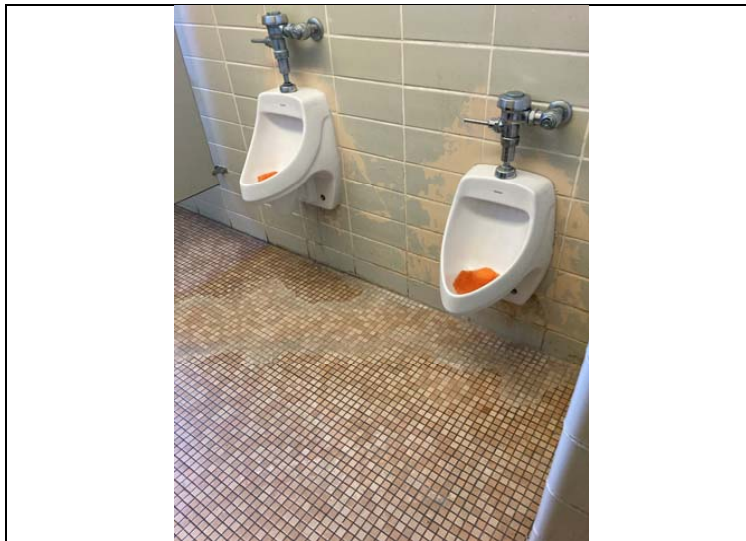
Bathroom Floor and Wall Tile
