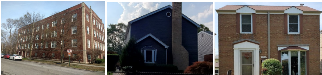
Building assessments will include single-family, two-flat, and small- to mid-sized multi-family buildings, like those shown here that were assessed during program design.
