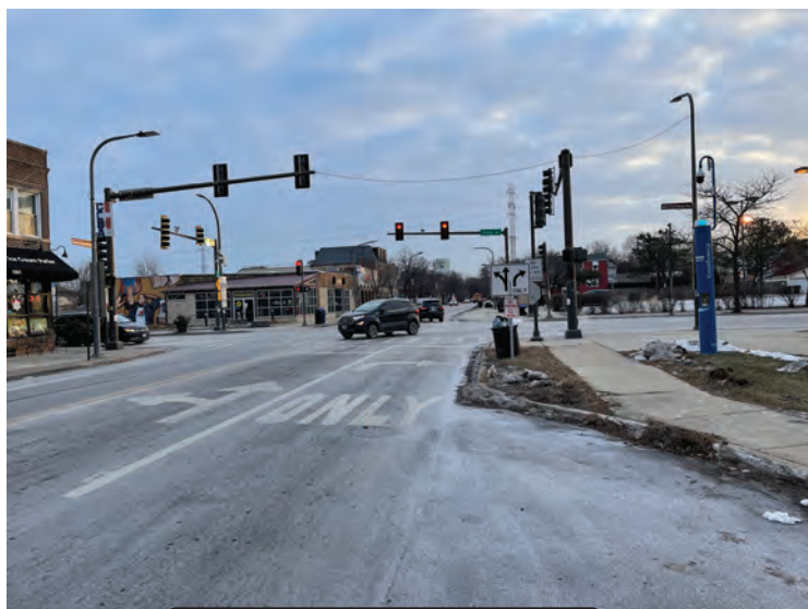
EASTBOUND APPROACH OF CHURCH ST / DODGE AVE INTERSECTION
