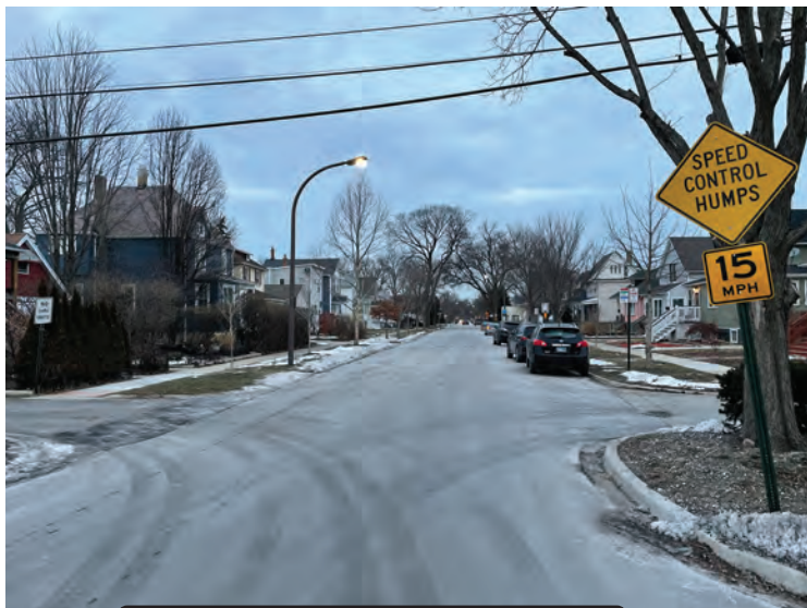
NORTHBOUND APPROACH OF DARROW AVE / CHURCH ALLEY INTERSECTION
