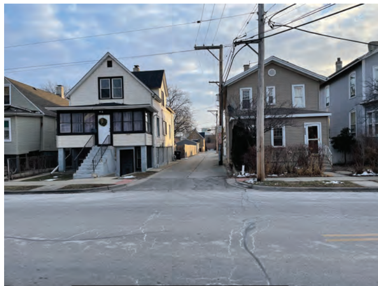
WESTBOUND APPROACH OF DODGE AVE / CHURCH ALLEY INTERSECTION
