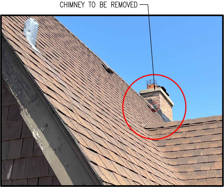
Photo of Ridge Chimney
