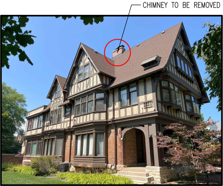
Photo of Ridge Chimney
