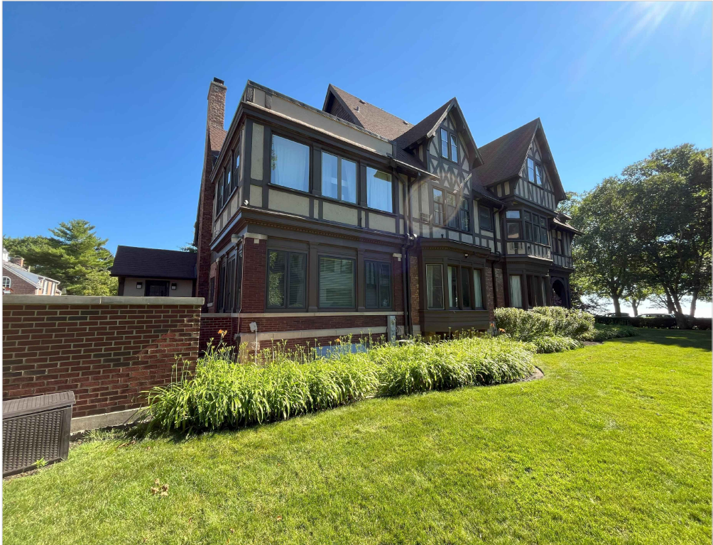
Photo of Deck Railing Looking North
